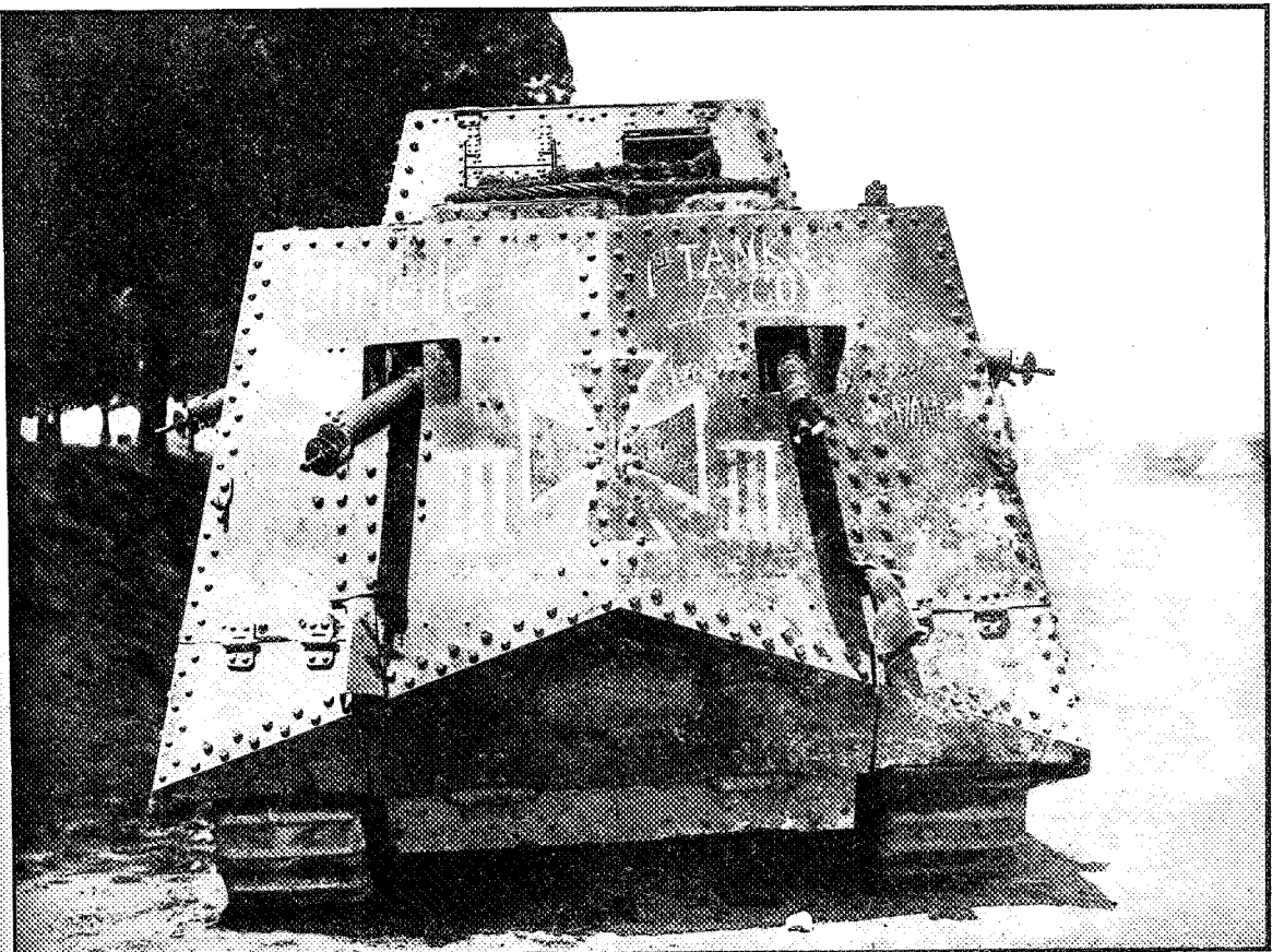
BACK VIEW OF THE TANK.
